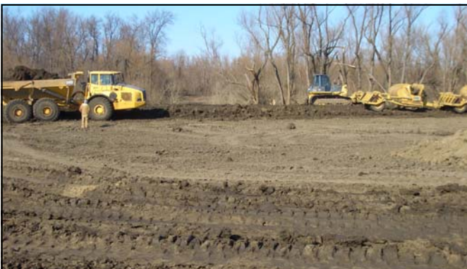
Repair of breached levees at Kings Lake. Photos by John Zimmerman
