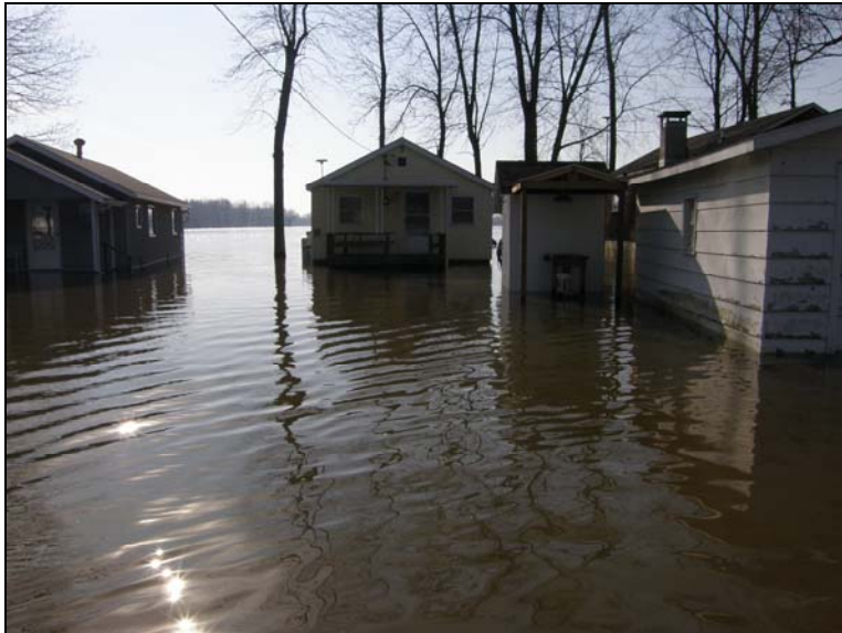
Figure 5-7. Waldron Lake – homes and accessory buildings surrounded by floodwaters in March 2009.
