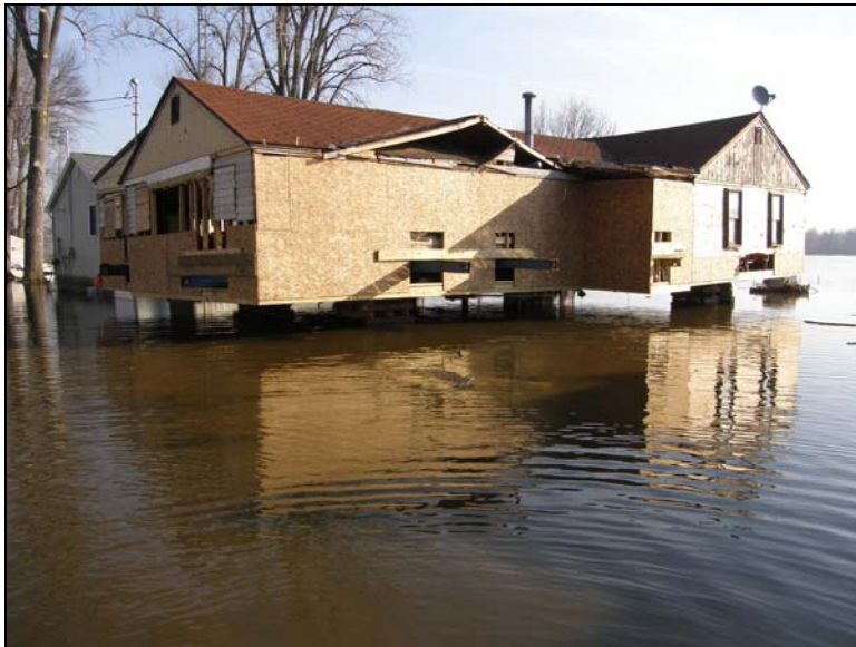
Figure 5-9. Waldron Lake – home damaged by 2008 flood in process of being repaired and elevated utilizing flood insurance/ICC in March 2009.
