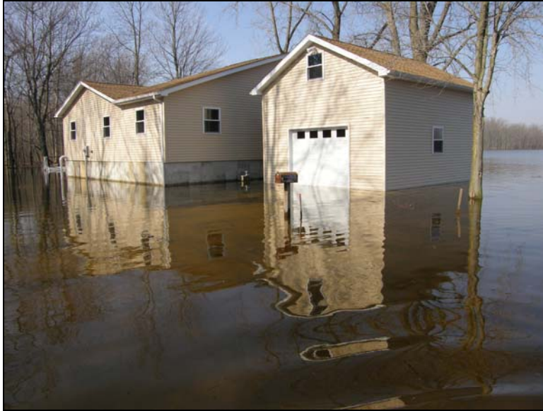
Figure 5-10. Waldron Lake – home damaged in 2008 repaired and elevated (stem wall construction), utilizing flood insurance/ICC undamaged in March 2009 flood.
