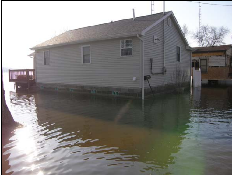
Figure 5-6. Waldron Lake – home damaged by 2008 flood repaired and elevated (enclosure beneath lowest floor with flood vents), utilizing flood insurance/ICC.
