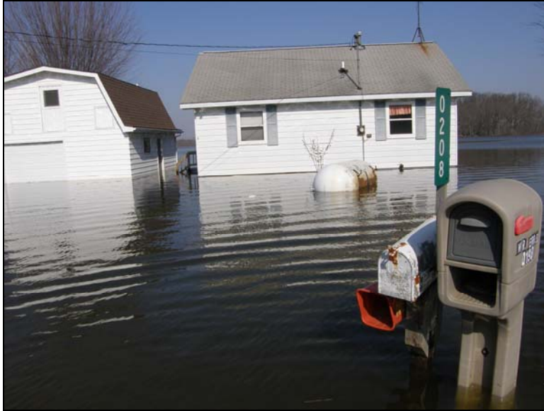
Figure 5-8. Waldron Lake – home with crawl space flooded and flooded garage in March 2009.
