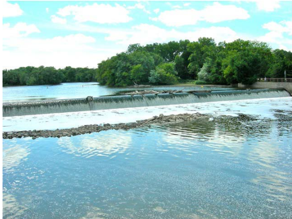
Low head dam in Illinois
