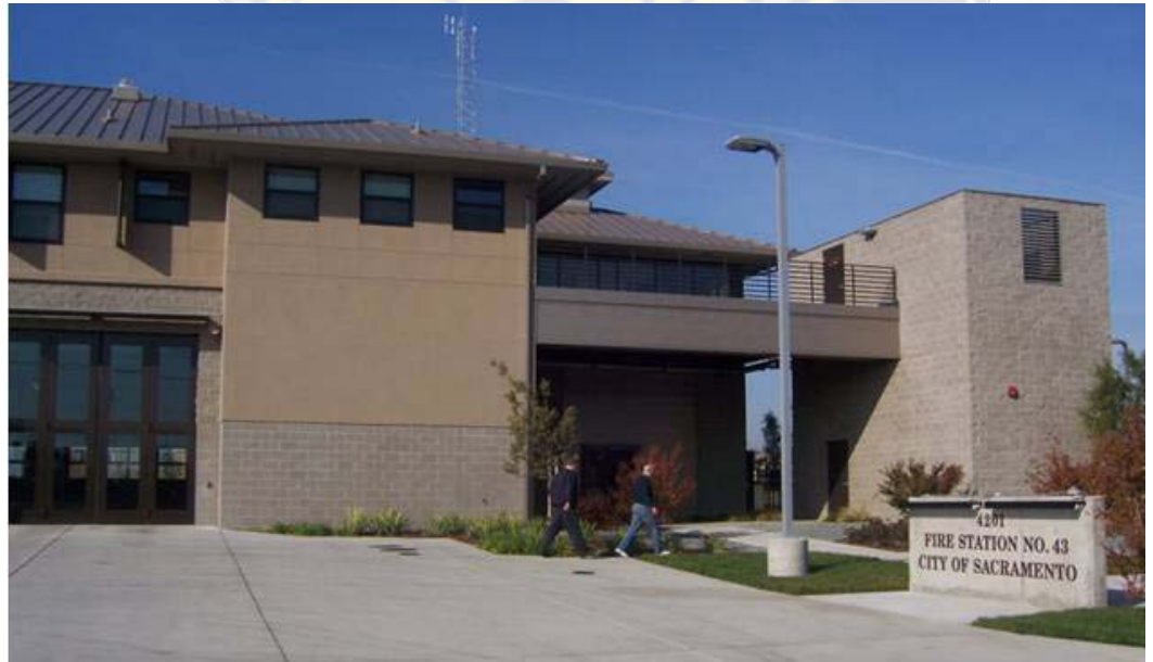
Natomas Fire station that has the second floor elevated above BFE.
